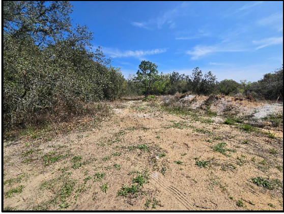
Photo 2.15. Cleared area with push pile within Pond 3B, facing east.
