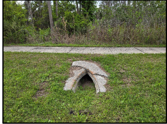
Photo 2.22. Example of concrete drainage along southbound Avalon Road, facing west.
