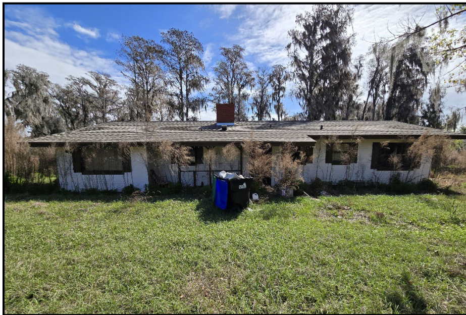
Photo 5.6. 14621 Avalon Road (8OR11764), looking east.
