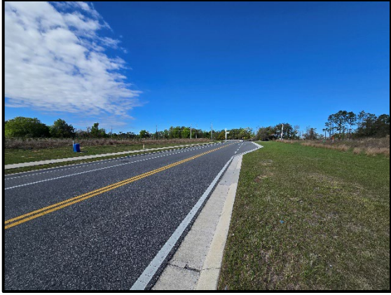
Photo 2.33. General conditions of Hartzog Road facing west towards Avalon Road.
